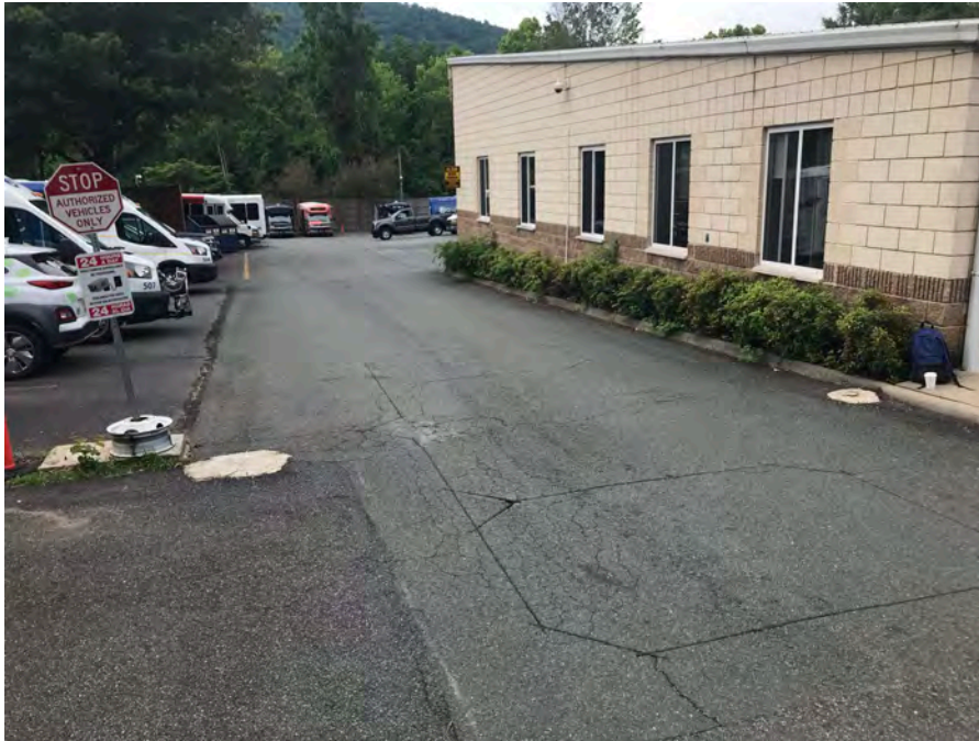
Figure 2. Looking South/Entrance to Maintenance Area
